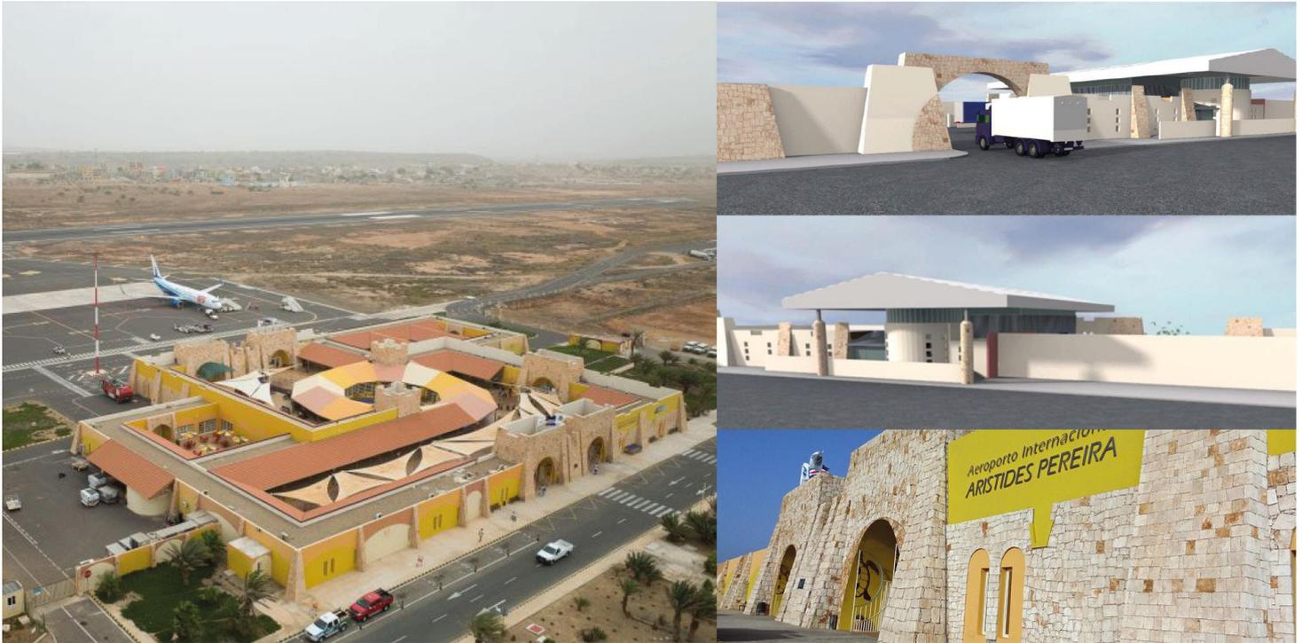
The new Cargo Terminal is formed by a perimeter wall built of concrete walls and rectangular concrete block walls enclosing a covered central area, which acts as a loading and unloading dock and offices, and two covered side areas for offices, maintenance and warehouse.
